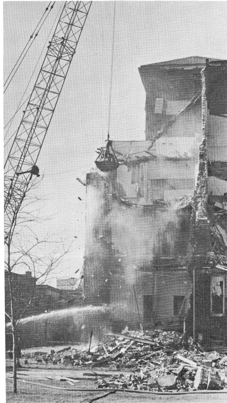
Old Main gives way to the wrecker's crane
